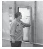
doors are prohibitive and discourage maintenance, which in turn can impact your operation. Specifying the size of the door will cause some bidders to take exception, alerting you to a potential maintenance headache. Two doors are standard on all Series Quiet towers—one in each endwall.
