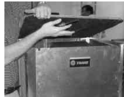
Step 12 Install unit top.
