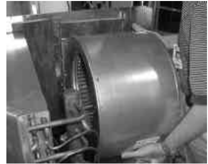
Step 9 Attach back panel with the blower motor assembly to the unit.
