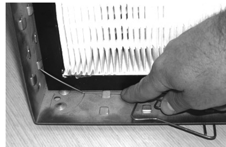
Figure 9. In order to remove the filters, unhook the clip which restrains the Final filter header within the UHF
