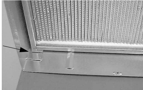
Figure 20. Once the HEPA is fully inserted into the AstroFrame, the latch holding slots should be clearly accessible at each of the corners
