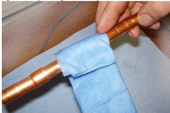
Figure 2. Wrap wet rag around the part
