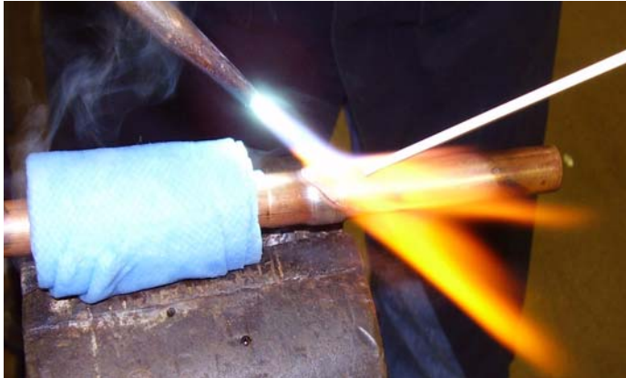
Figure 5. Always direct heat away from delicate parts.
