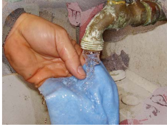
Figure 1. Apply water to rag that will be used to keep part cool.
