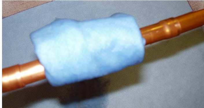
Figure 3. Wrap wet rag around part completely, leaving joints exposed
