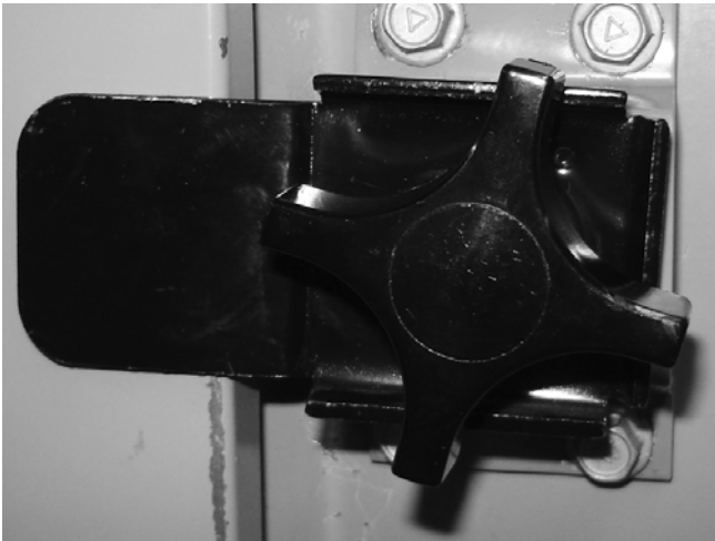
Figure 6. Completed installation of latch assembly
