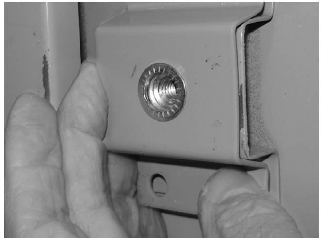
Figure 4. Placing new bracket over existing bracket
