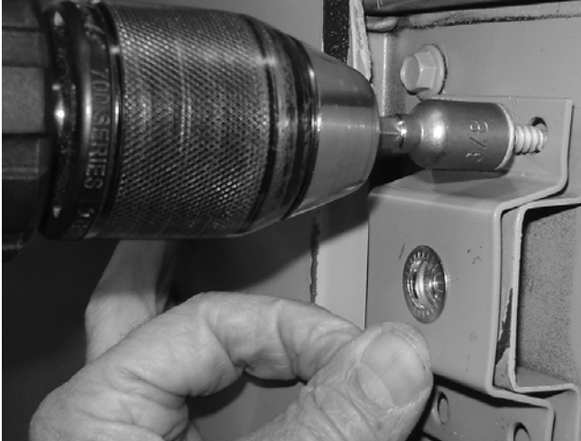
Figure 5. Securing new latch bracket
