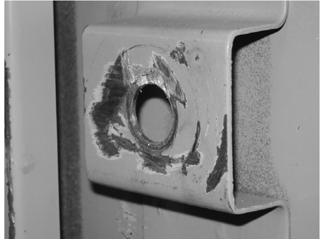
Figure 3. Completed removal of rivet nut
