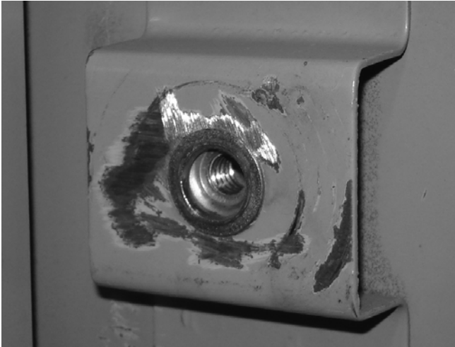
Figure 1. Removal of existing latch
