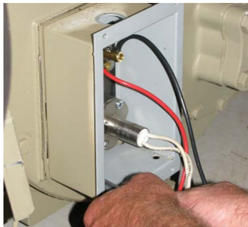
Figure 10. Reinstalled terminal box
