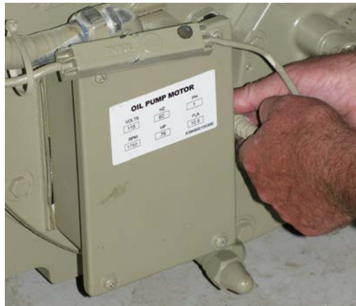
Figure 11. Connect power
