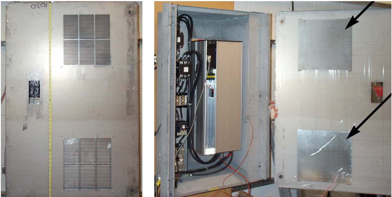
Figure 1. Remove existing louver baffles
