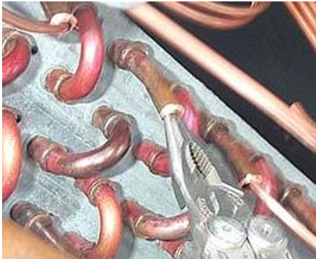
Figure 5. Bringing tubes back to round
