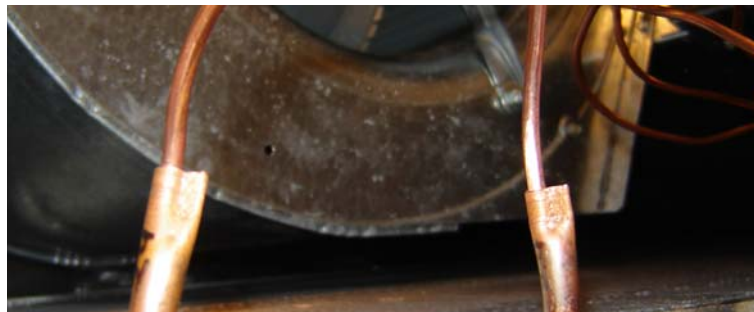
Figure 8. Distribution tubes crimped into place
