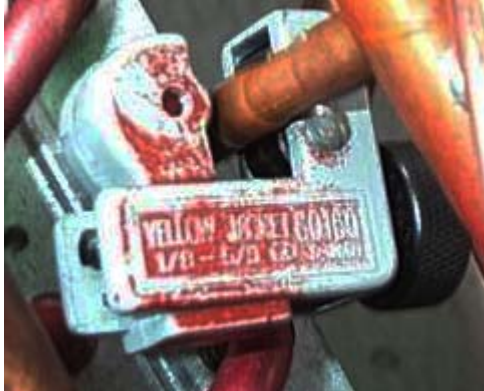
Figure 4. Cutting tubes just below the existing orifice
