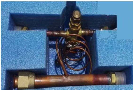
Figure 10. Thermostatic Expansion Valve TXV
