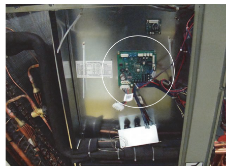
Figure 12. RTOM board in T/YSC120 unit
