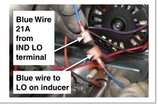
The inducer and all associated wires should now be connected.
