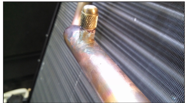
Figure 14 – Sealed Schrader core
