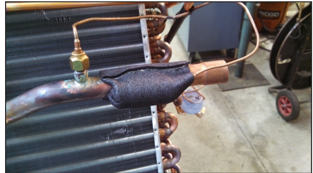
Figure 19 – Insulating the sensing bulb
