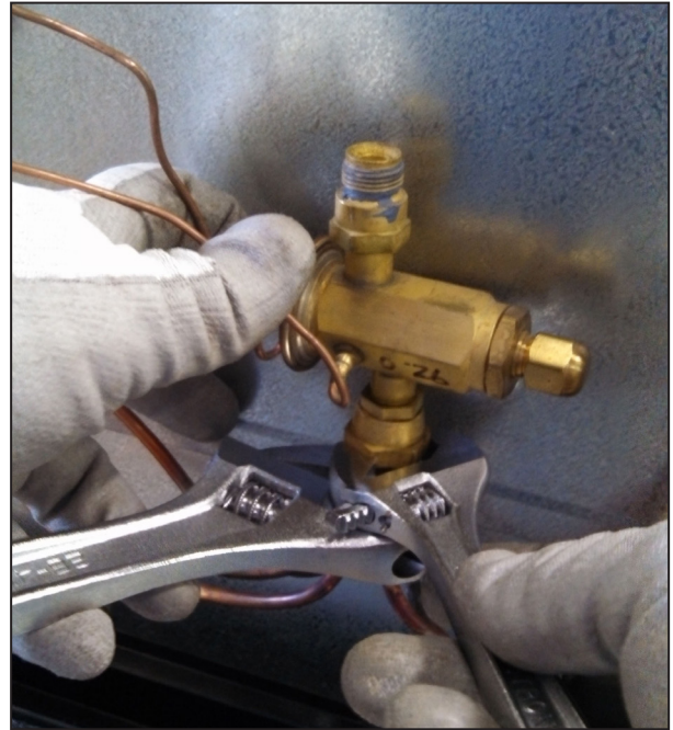
Figure 5 – Installing TEV
