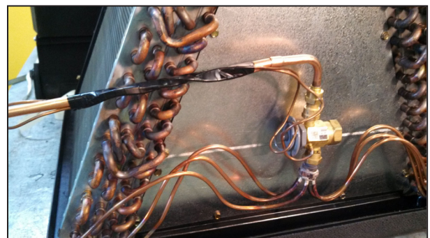
Figure 15 – Wrapping liquid line
