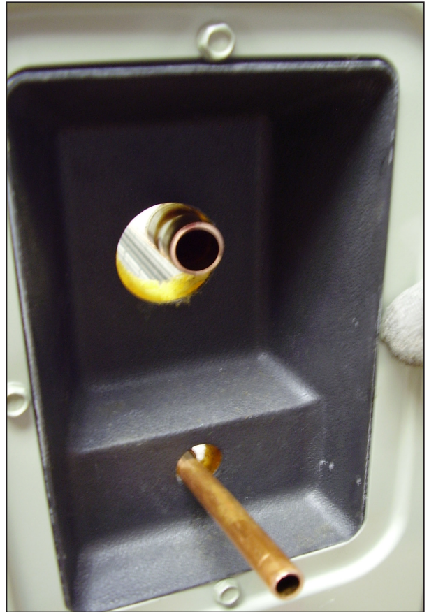
Figure 17 – Routing lines through panel
