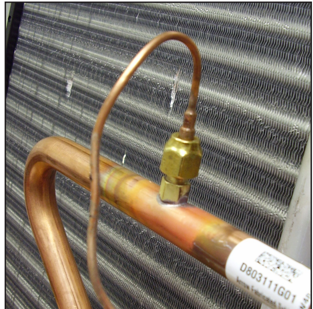
Figure 9 - Connecting equalizer line
