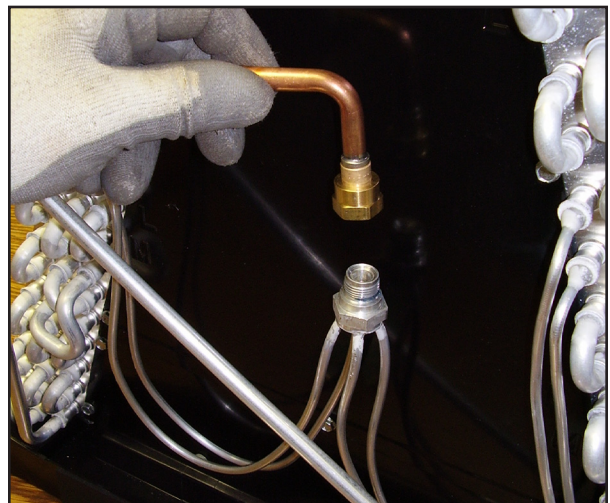
Figure 4 - Removing short liquid line
