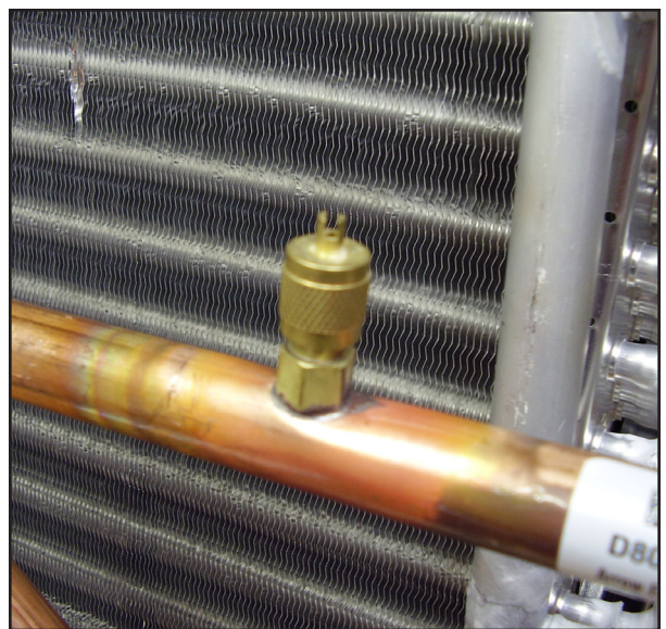
Figure 14 - Sealed Schrader core
