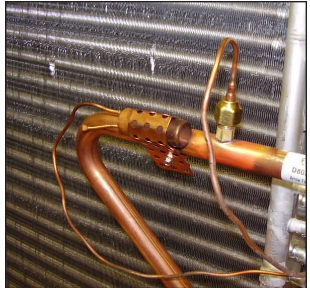
Figure 18 - Attaching sensing bulb
