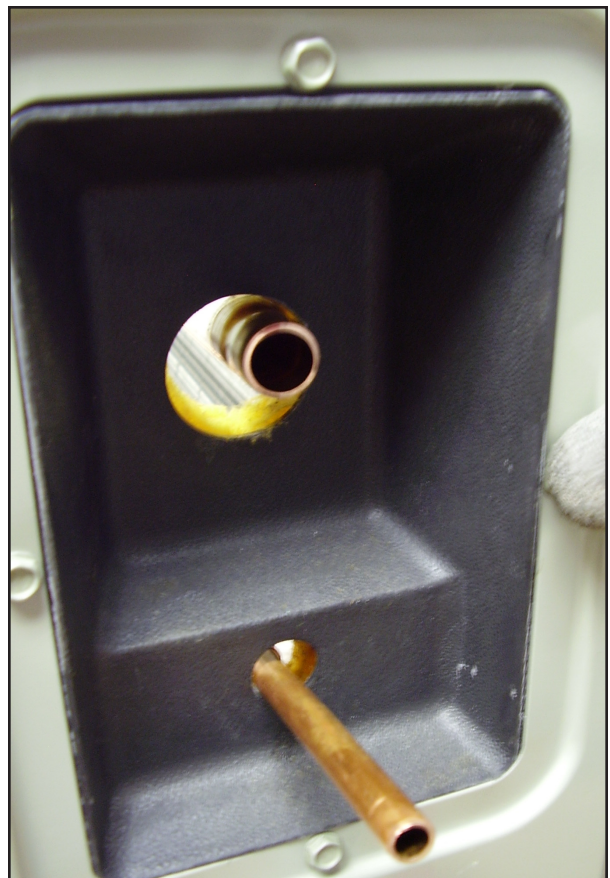
Figure 17 - Routing lines through panel
