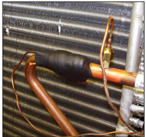
Figure 19 - Insulating the sensing bulb
