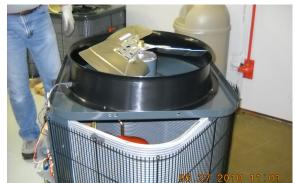
Mark the orifice ring and top panel with a reference mark before removing the orifice ring from the top panel.
