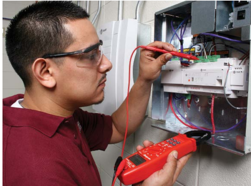
Trane-equipped HVAC lab, Gateway Technical College - Kenosha, Wisconsin; founding member of NC3
