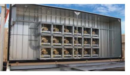
*Direct-Drive Plenum (DDP) fan arrays allow up to 100 percent redundancy for greater systems reliability and up to 10 percent increased efficiency.*
