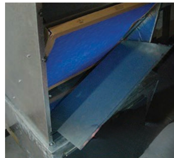
Figure 9. Bottom return application
