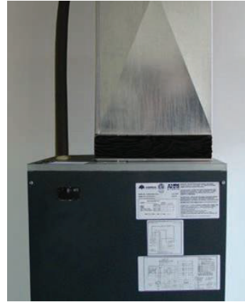
Figure 8. Prevent transmission of vibration
