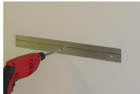
Figure 13. Pilot holes
