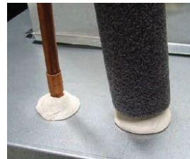
Figure 31. Seal the openings
