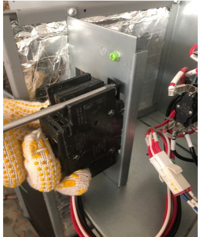
Figure 7. Install breaker
