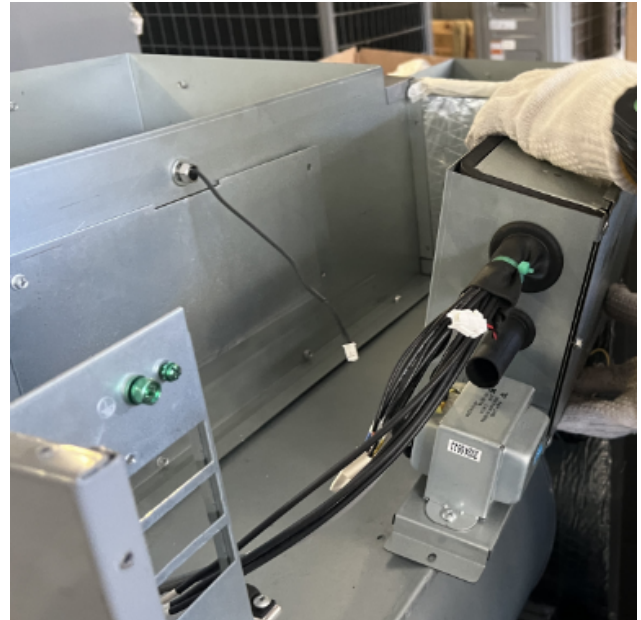
Figure 3. Remove electrical box
