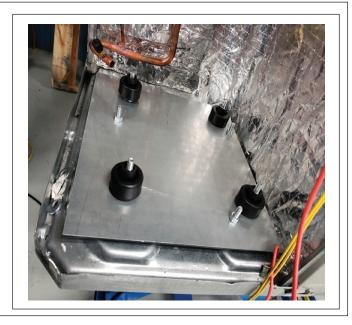
**STEP 4** -After securing the compressor to the mounting plate using new grommets and screws, slide the crankcase heater around the compressor, tighten the mounting screw and secure the wires out of the area that you will be brazing.
