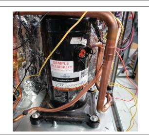
**STEP 6** - Braze, leak check with nitrogen, vacuum and recharge per data plate.
