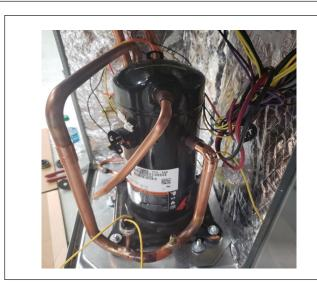
**STEP 7** - Install new compressor power lead, LPCO wires, connect crankcase heater wires and secure any other wires that were moved during the compressor replacement. Replace run capacitor if required in parts notes.
