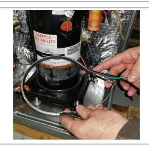
**STEP 5** - Set the new compressor, tighten the mounting nuts and use the Trane-supplied tubing connectors to dry-fit the pipes before brazing. Replace liquid line drier in the outdoor coil section of the unit.
