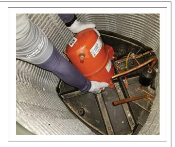
**STEP 3** - On heat pump units only, install the sump heater prior to setting the new compressor inside of the unit.
