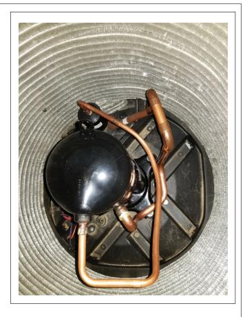
**STEP 6** - Install new compressor power leads, connect crankcase heater wires (heat pump only), reconnect LPCO wires, and secure any other wires that were moved during the compressor replacement. Replace run capacitor if required in parts notes. Run-test system for proper operation.
