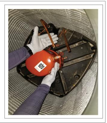
STEP 2 - Remove the compressor from the unit.
