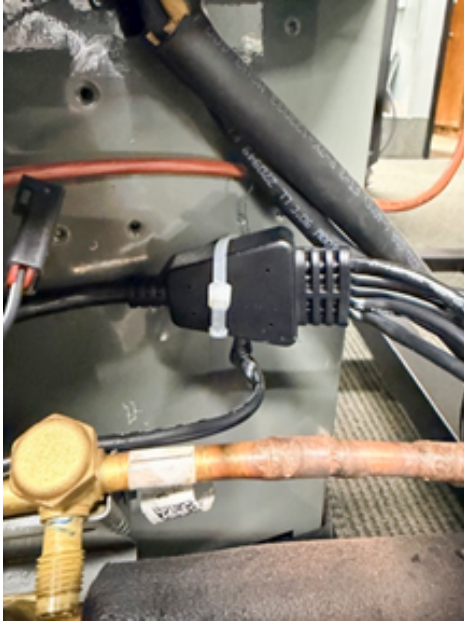
Figure 9. Install the outdoor harness
