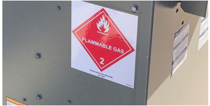
Trane units containing A2L refrigerants will include a Class 2.1 Flammable Gas label.
