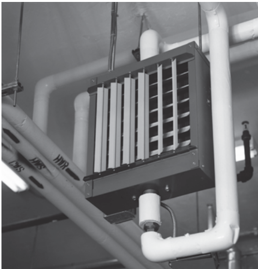
Figure 2. Model S horizontal unit heater, header type (with optional vertical louver kit installed)
