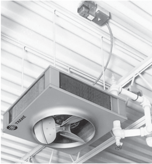
Figure 2. Model S horizontal unit heater, header type (with optional vertical louver kit installed)
