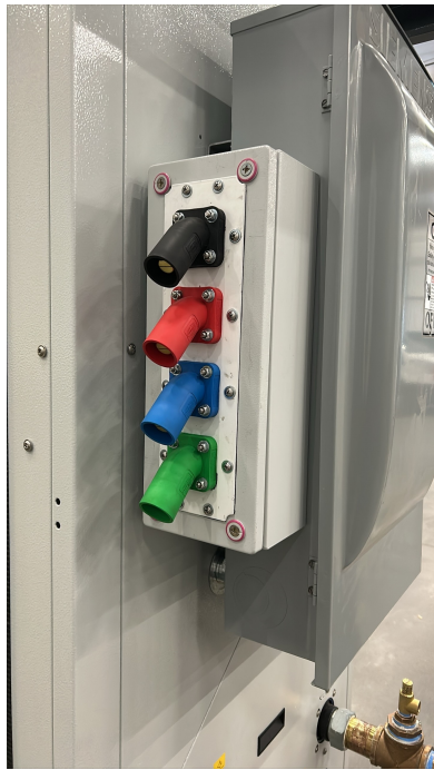
Figure 19. 3-15 Ton Pin and Sleeve Power Connection
