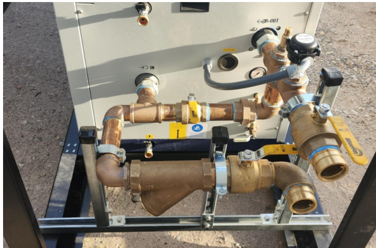
Figure 23. Victaulic water connections for 20 and 40 ton models
