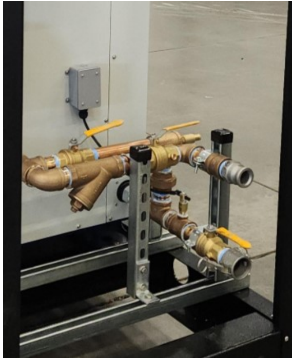
Figure 22. Cam-lock water connections for 3 —15 ton models
