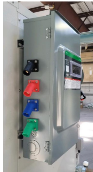
Figure 25. MTA unit mounted fused disconnect with pin & sleeve power supply connections
