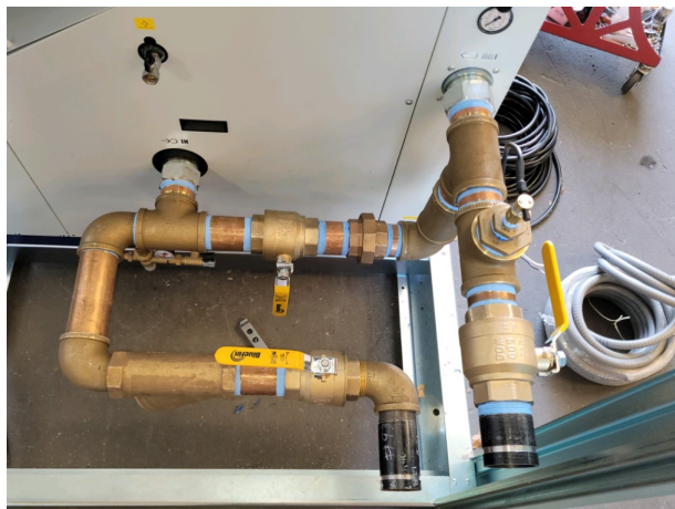
Figure 29. Victaulic water connections for 20 and 40 ton models
