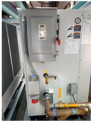
Figure 25. MTA unit mounted fused disconnect with pin & sleeve power supply connections
