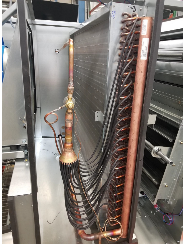
Figure 13. Evaporator coil
