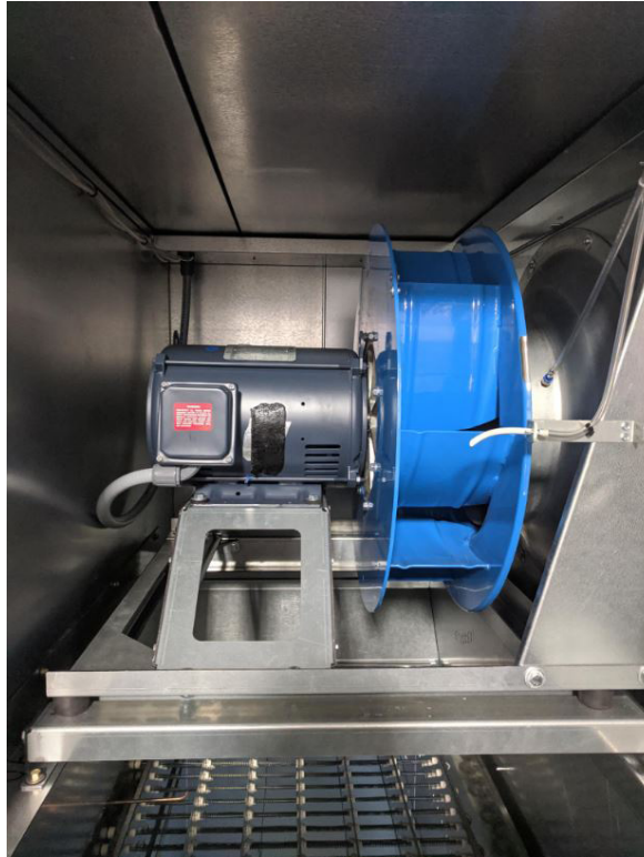
Figure 16. Supply Fan
