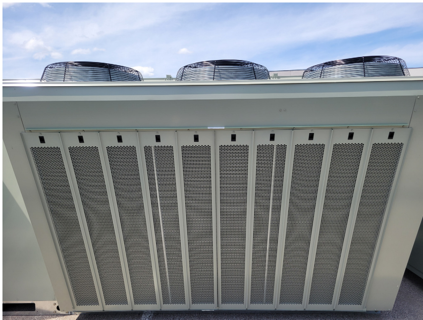
Figure 88. Condenser hail guards
