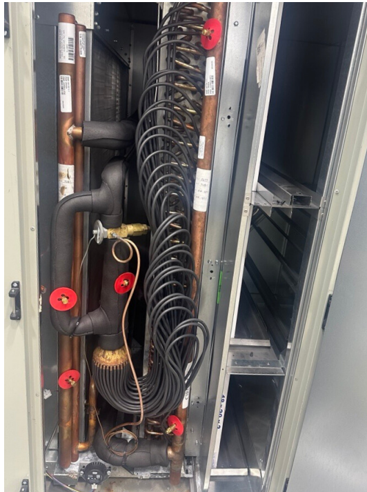
Figure 80. Evaporator and reheat coil
