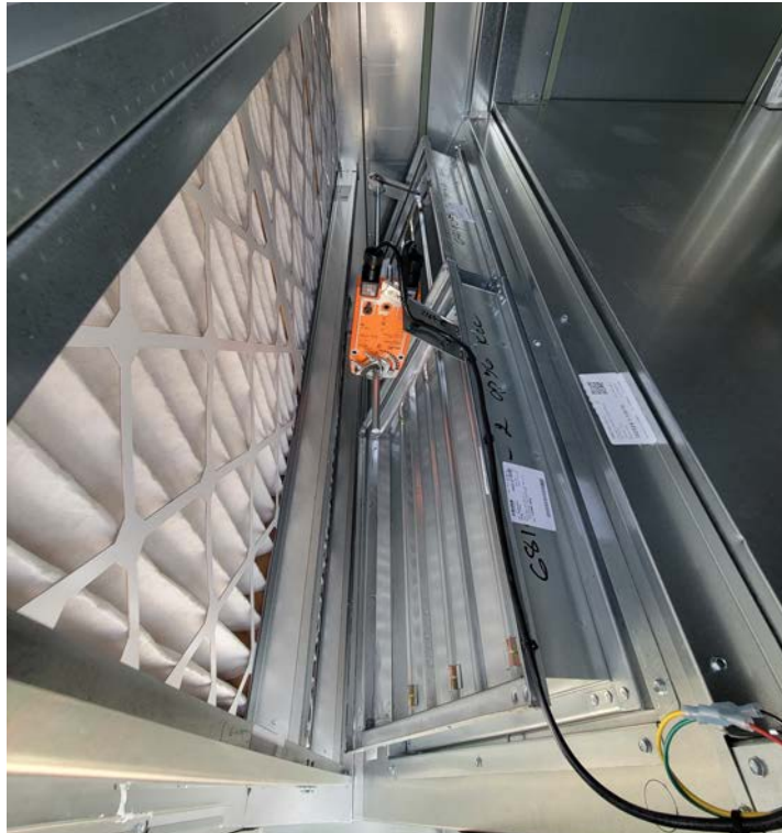
Figure 84. Return air damper
