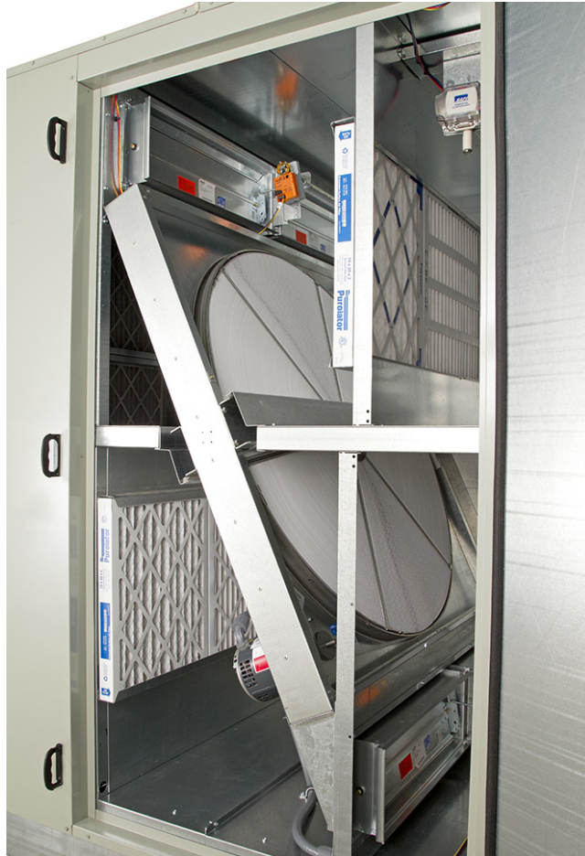
Figure 81. Total-energy wheel module
