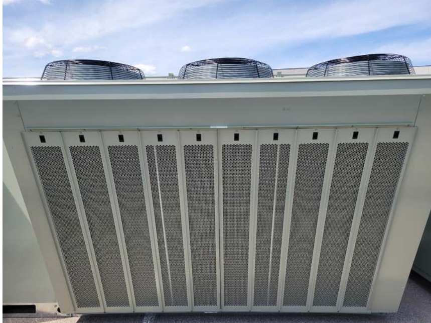
Figure 87. Condenser hail guards
