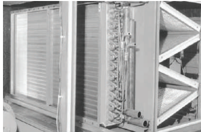
Figure 3. Cooling coils
