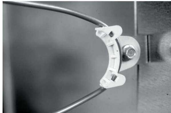
Figure 3. Factory-mounting ensures quality installation, as shown with the low-limit radius bend
