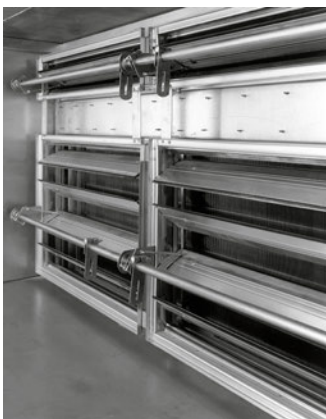
Figure 39. Internal dampers
