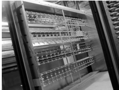
Figure 36. Typical blow through heater
