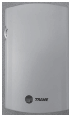
Figure 18. Wall-mounted fan speed switch (Digit 38 = F)
