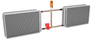
Coil loops, sometimes called coil run-around loops, have two or more finned tube coils that are piped together in a closed loop. A fluid is circulated by a pump between the coils to transfer sensible heat from one air stream to another. The fluid is often water mixed with a freeze inhibitor like glycol.
