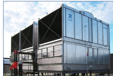
Closed-circuit cooling tower "fluid cooler"
