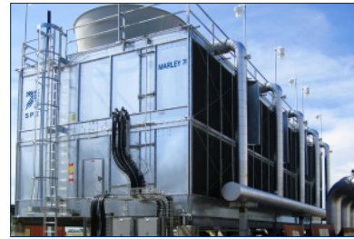
Open-circuit cooling tower
