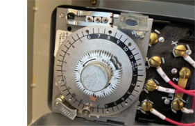
Figure 8. Setting the defrost timer
