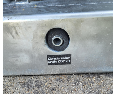
Figure 1. Condensate drain
