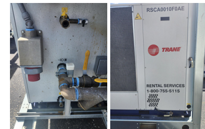
Figure 5. Vent valves - TRS modified unit
