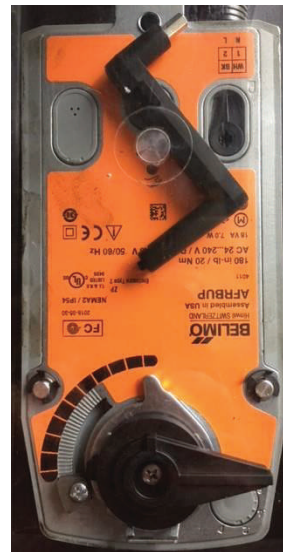
Figure 6. Powered open position (cooling cycle)
