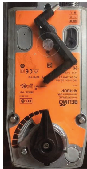
Figure 6. Powered open position (cooling cycle)
