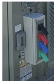
Figure 4. Cam connectors
