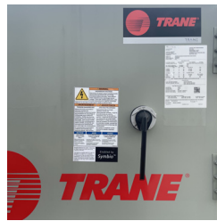
Figure 5. Unit disconnect
