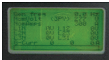
Voltage Readout: To read this screen, press the ▼ button. Monitor L12, L23, and L31 while adjusting voltage
