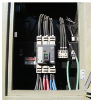
Access to Breaker, Terminal Blocks, Shore Power Connection, and Remote Engine Start Contacts Never Open While in Operation
