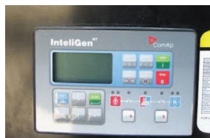
Digital Controller Use the Mode button to select OFF, MAN, or AUTO mode Use the Up or Down button to access diagnostic screens (fuel level, oil pressure, engine temp, etc.)
