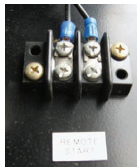
Remote Engine Start Contacts
