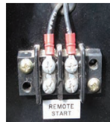
Remote Engine Start Contacts
