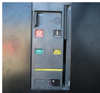
Circuit Breaker Do Not Use Manual Push Buttons
