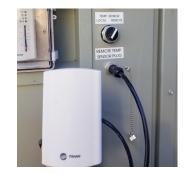
4. Wire incoming electrical cable into pin, cam-type connections and outgoing cable to sleeve, cam-type connections. If equipped with and outgoing connections are not to be used, use bar to Lock Out, Tag Out sleeve connections
