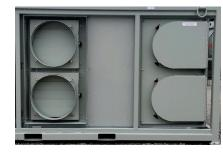
If needed, connect the remote sensor (inside the return air cabinet) to quick connect and adjust sensor selector switch accordingly (above quick connect on the front of the machine).
