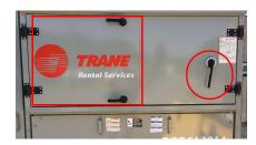
On the Mode Control Panel, verify power on light is ON and phase failure light is OFF.
