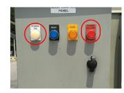
8. Verify system switch is in the **ON** position on the Mode Control Panel.
