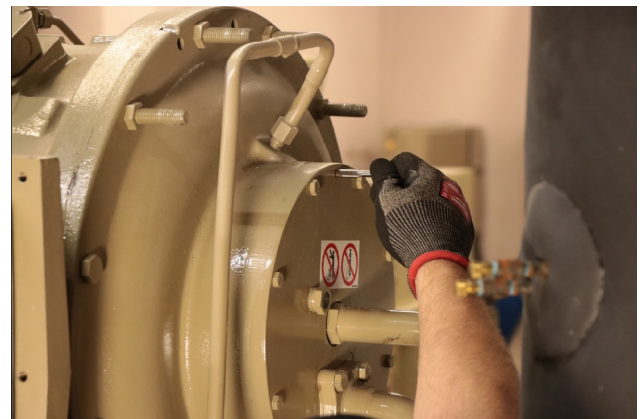
Figure 5. Cleaning motor plate threads
