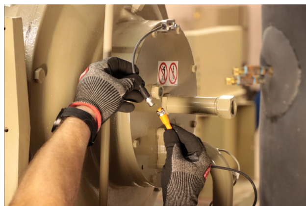
Figure 18. Connect sensor wire
