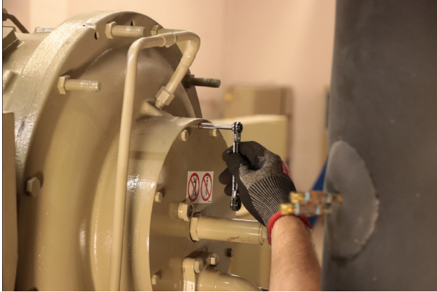
Figure 6. Ratchet wrench cleaning
