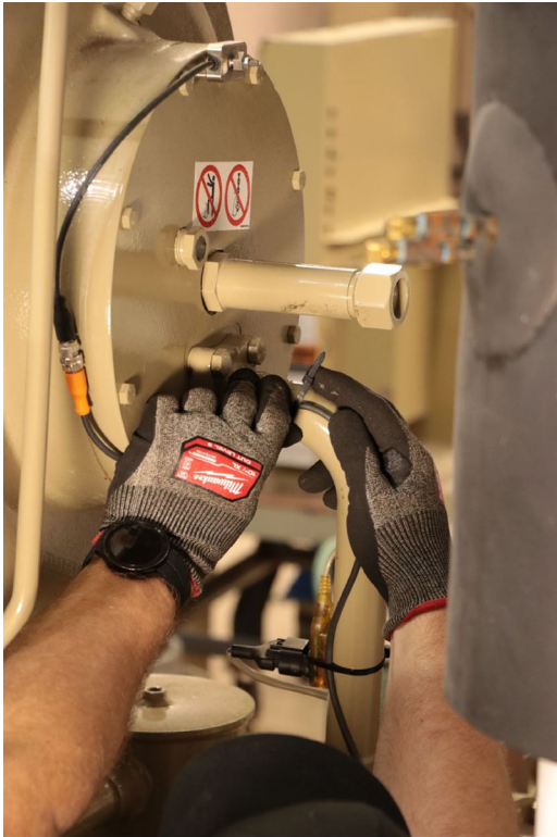
Figure 19. Lock sensor wire into position
