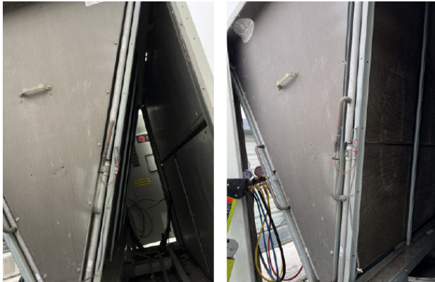
Figure 21. Thermistor sensor on condenser coils (MCHC coil) location
