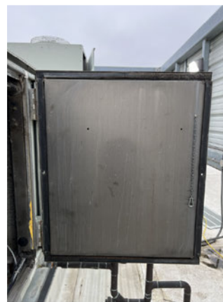
Figure 12. Gasket and screws for access doors and panels location
