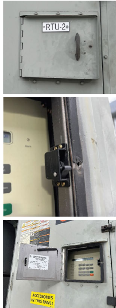
Figure 23. Control panel handle and latch location
