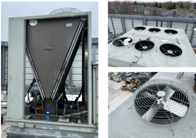
Figure 43. Condenser coil, and fan guard locations
