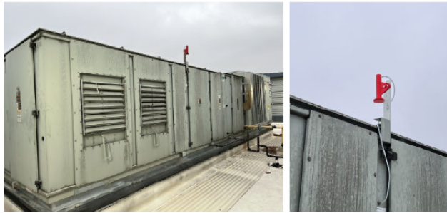
Figure 14. Outside air static pressure sensor kit location
