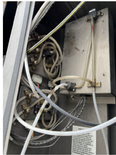
Figure 49. Air pressure sensor kit location
