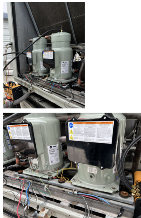
Figure 32. Compressor and related parts
