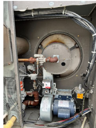
Figure 47. Gas heat exchanger, motor, limit control, and electric heater
