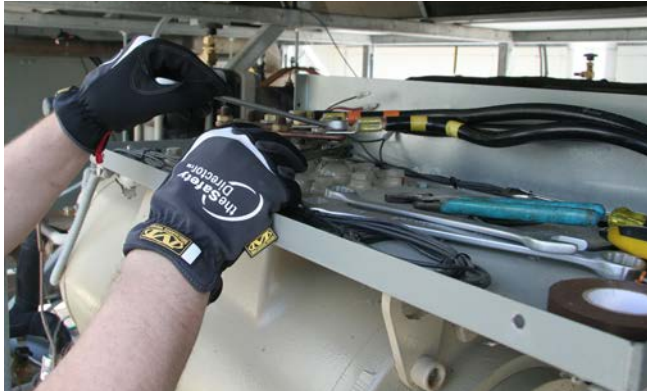
Figure 57. Connect wires to motor terminals
