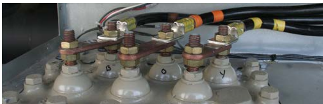
Figure 58. Install shorting bars for wye-delta starters
