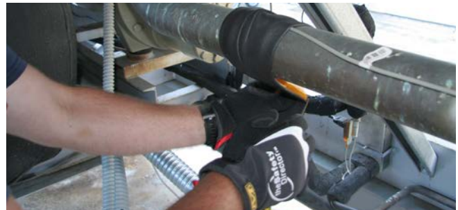
Figure 66. Sensor covered with insulating tape
