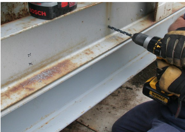
Figure 14. Drill 5/8-inch holes in base
