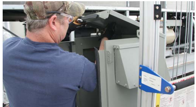
Figure 21. Remove top cover of enclosure
