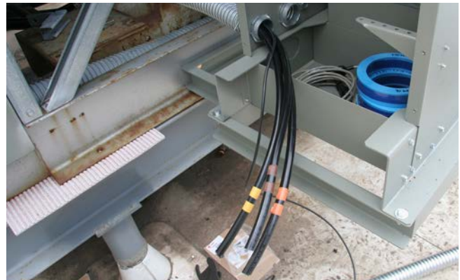
Figure 45. Install conduit at AFD enclosure
