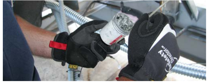
Figure 64. Use thermal paste on sensor
