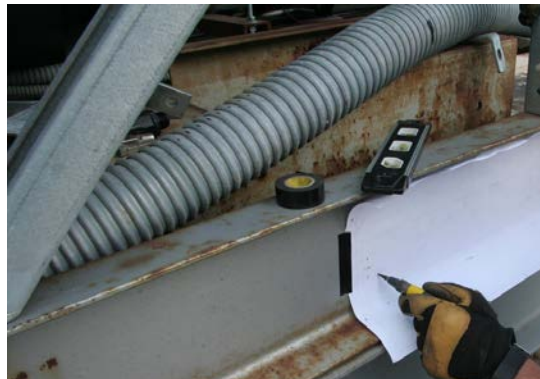
Figure 12. Mark drilling locations with template
