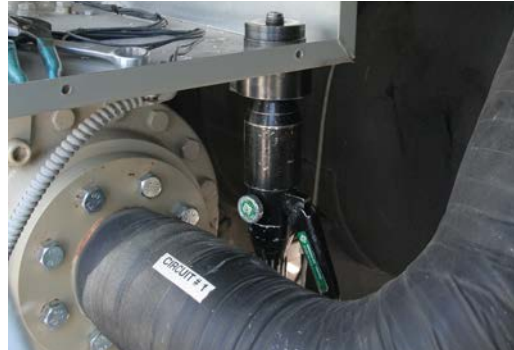
Figure 54. Create compressor conduit connection point
