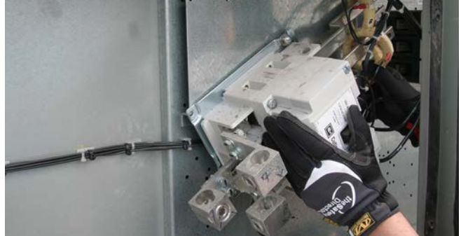
Figure 36. Contactor left in place
