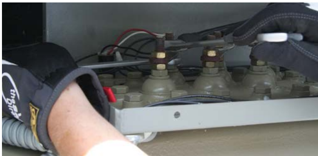
Figure 53. Remove compressor wiring
