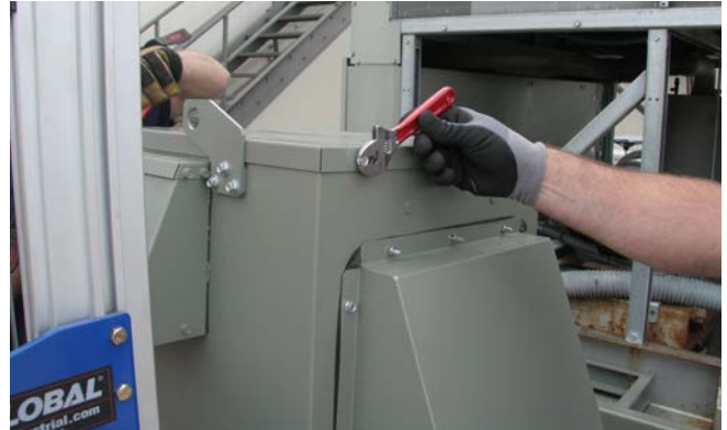
Figure 21. Remove top cover of enclosure
