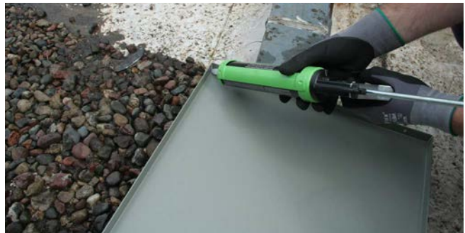
Figure 30. Apply caulk
