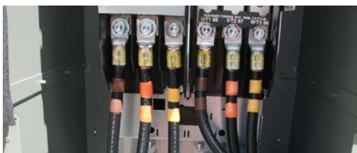
Figure 48. Install output wire at AFD
