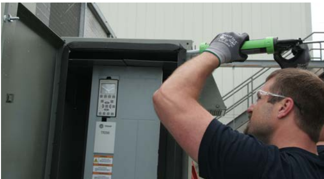
Figure 33. Apply sealant
