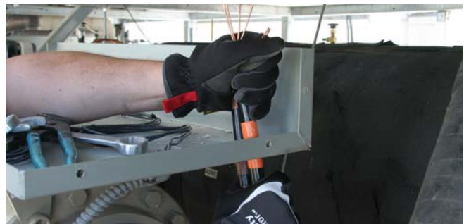
Figure 56. Install conduit at compressor
