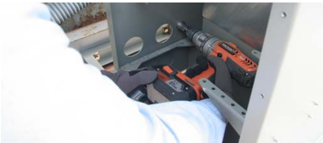
Figure 44. Create AFD conduit connection
