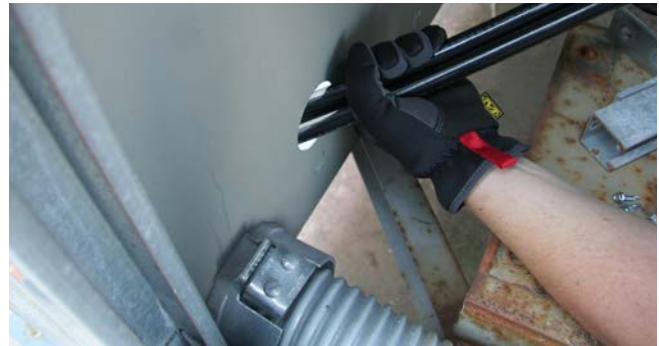
Figure 42. Route power wire to AFD
