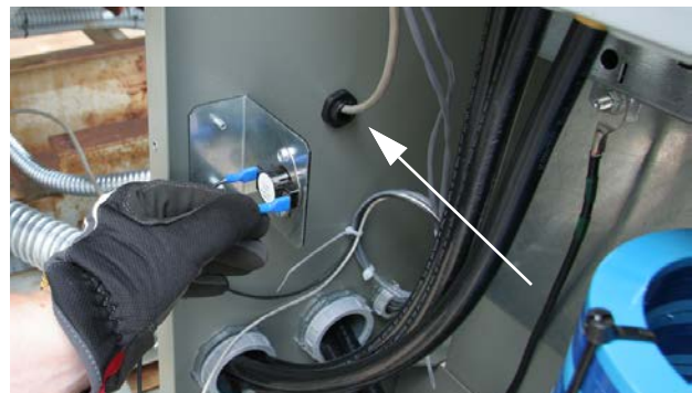
Figure 62. Global connector wires
