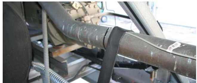
Figure 66. Sensor covered with insulating tape
