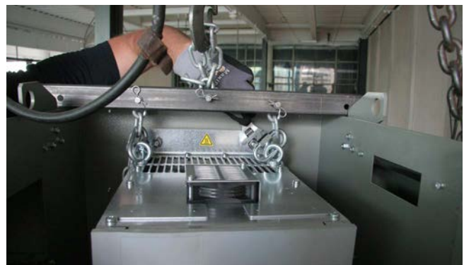
Figure 25. Install on mounting studs
