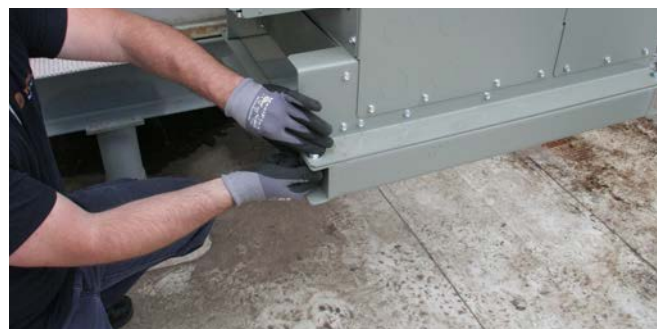
Figure 16. Attach enclosure to mount
