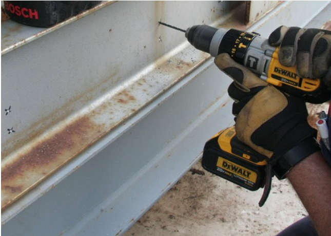
Figure 14. Drill 5/8-inch holes in base
