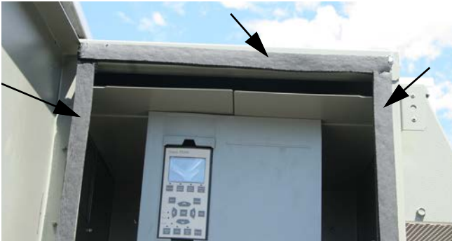
Figure 31. Gasket installed
