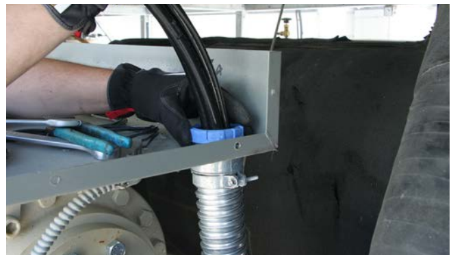
Figure 56. Install conduit at compressor
