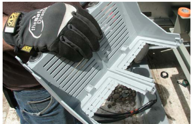
Figure 52. Touch safe cover installed
