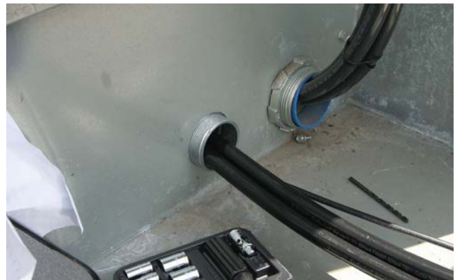
Figure 42. Route power wire to AFD
