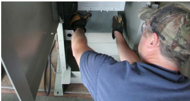
Figure 19. Remove bottom airflow duct
