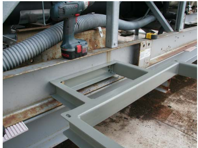
Figure 15. Mounting bracket installation
