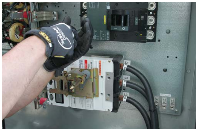
Figure 37. Install circuit breaker
