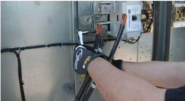
Figure 34. Remove compressor wire
