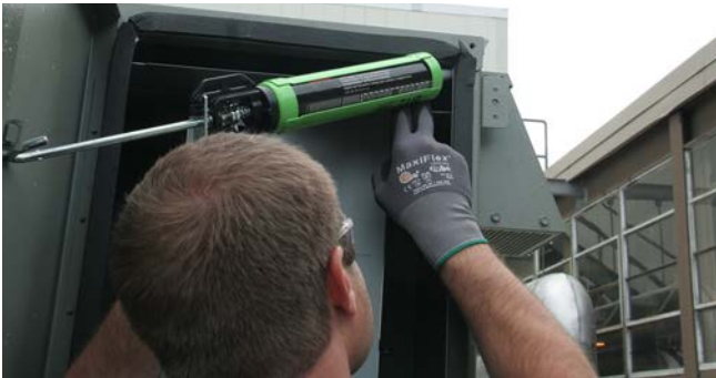
Figure 32. Apply sealant
