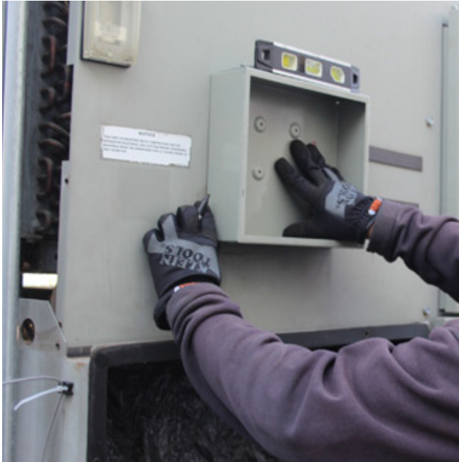
Figure 8. Leveling enclosure and hole marking
