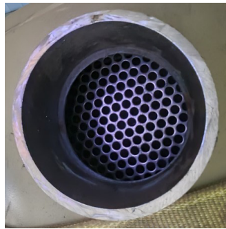
Figure 48. Perforated plate on inlet
