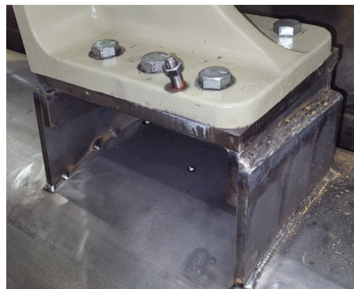
Figure 28. Compressor base finish weld
