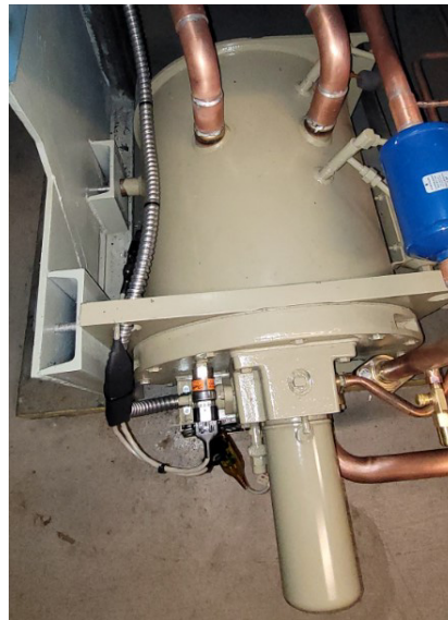
Figure 17. Tank assembly support
