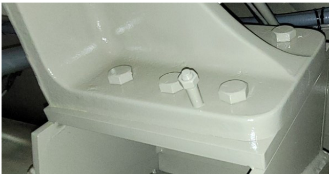
Figure 6. Compressor foot dowel pin
