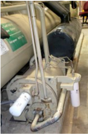
Figure 14. Tank in-line with economizer – rigging ear trimmed
