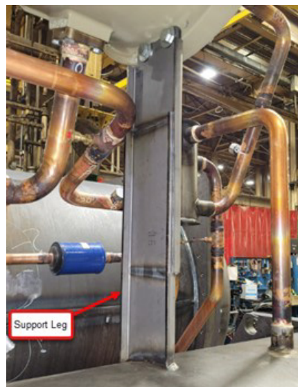
Figure 30. Compressor support leg
