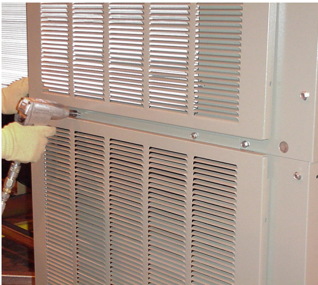
Figure 6. Top and bottom panels installed
