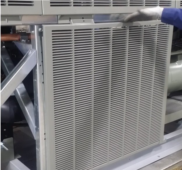
Figure 6. Top and bottom panels installed
