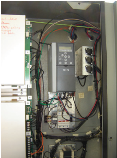
Figure 6. Mounted drive assembly
