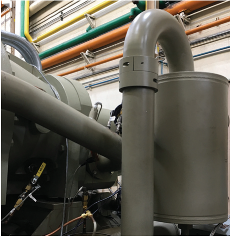
Figure 29. Line weight installation location – B-frame compressors
