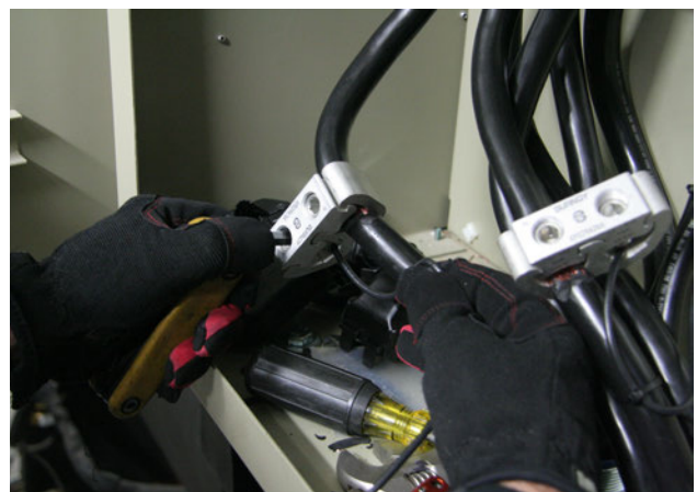
Figure 69. 12 AWG wire connections
