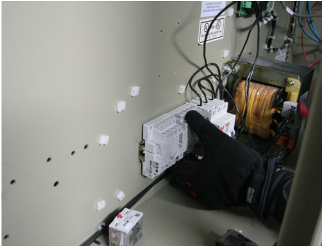
Figure 43. 1K1, 1K2 relay socket
