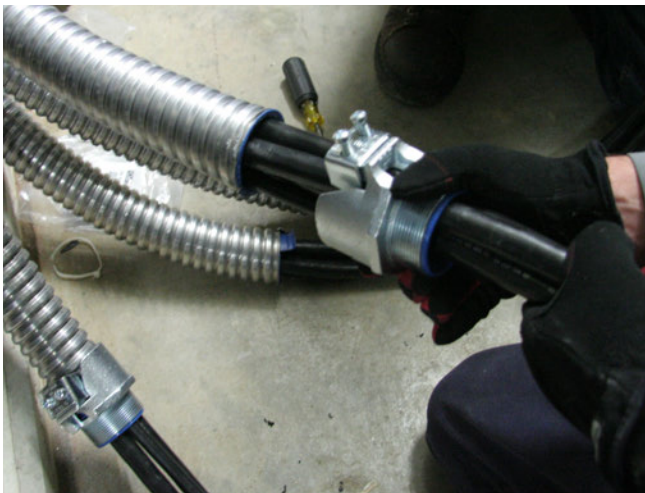
Figure 50. Conduit connector assembly
