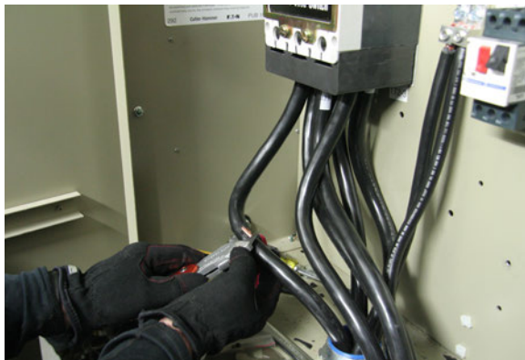
Figure 68. Wire tap installation
