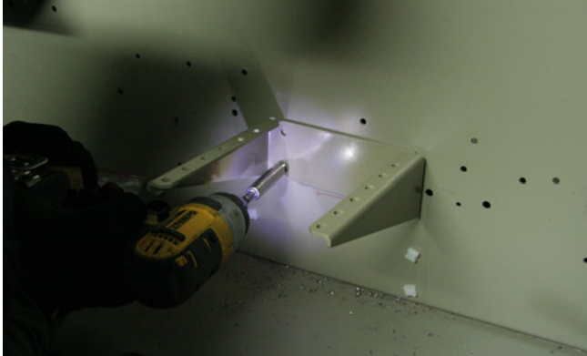
Figure 39. Choke core support bracket
