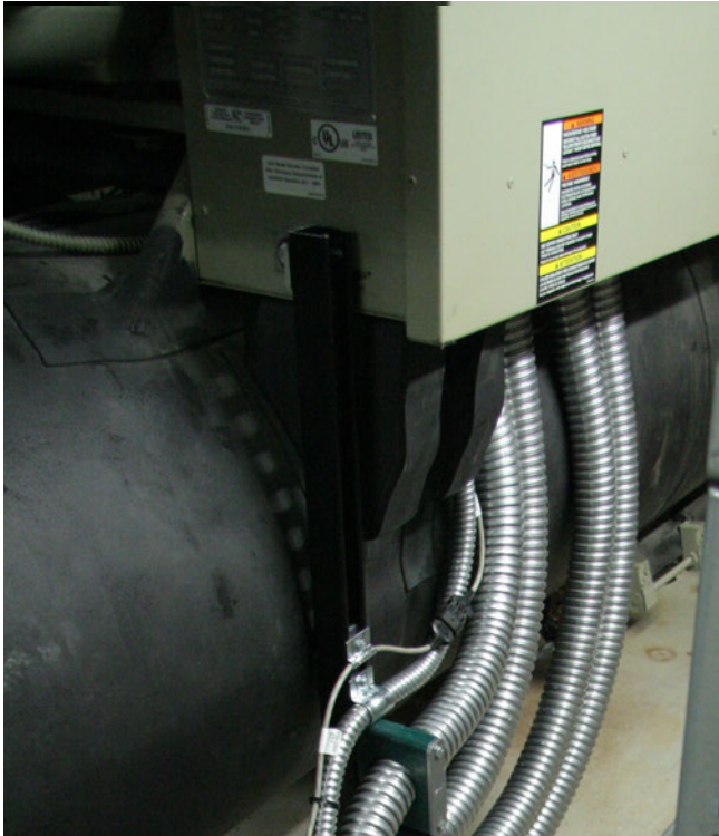
Figure 50. Conduit connector assembly
