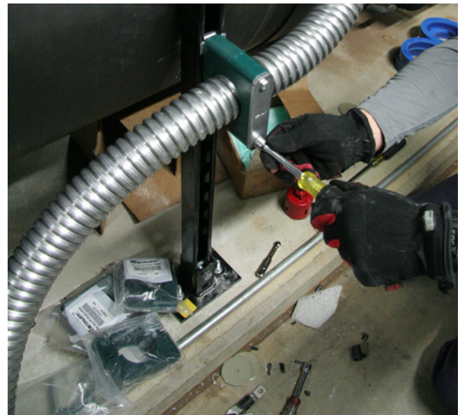
Figure 52. Power wire conduit mounting
