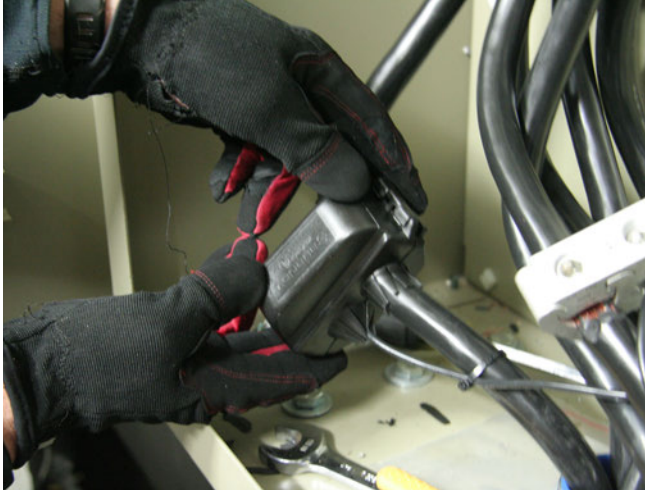
Figure 70. Wire tap case install
